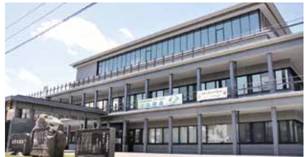
災害対策本部(市庁舎) Headquarters for emergency disaster control (City Hall) 灾害对策总部(市政厅)
