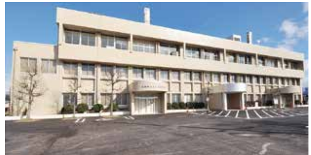
災害時医療拠点(休日急患診療所) Medical center at the time of disaster (holiday emergency clinic) 灾难医疗中心(假日急诊)
