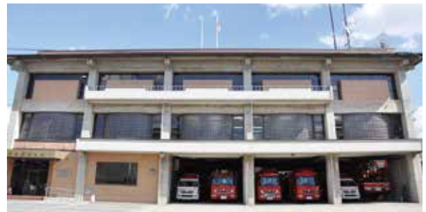
消防本部(消防署) Fire-Fighting Headquarters (Fire-Fighting Department) 消防总部(消防部门)
